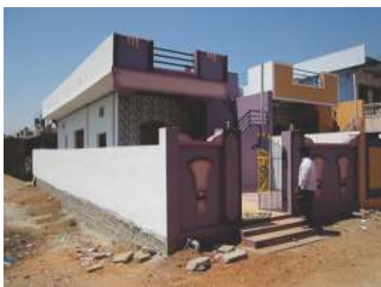
Kodumur Village, Karnool District (A.P.)
