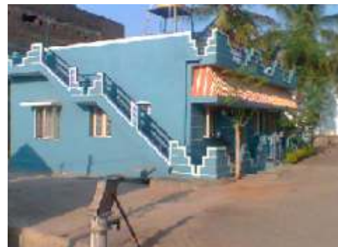
Kollegal, Chamrajnagar, Mysore, Karnataka.
